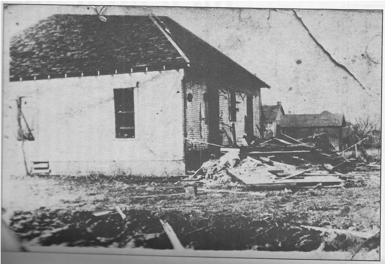
Figure 24: The home of O.M. Lamb, the undersheriff in 1921. The porch was destroyed by dynamite, and windows up to a mile away from the home broke with the impact of the explosion. This was the second time Lamb had been targeted by bootleggers in January 1921. Source: Kansas Bootleggers.
