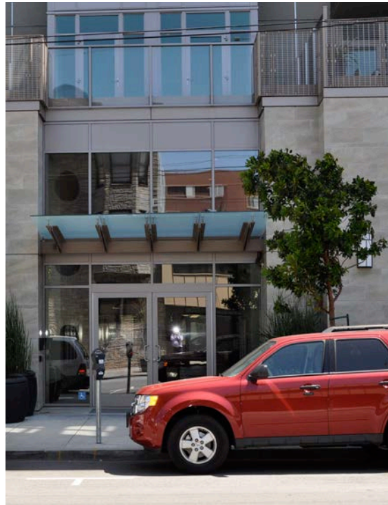
Wide, high and transparent doorways which are set back and combined with projecting awnings create protected, inviting, and identifiable entries to a building.
