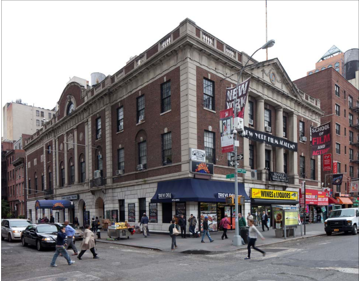
Tammany Hall 100 East 17 th Street, (aka 100-102 East 17 th Street, 44-48 Union Square, 44-48 Union Square East) Borough of Manhattan Tax Map Block 872, Lot 78 Photo: Christopher D. Brazee, 2013
